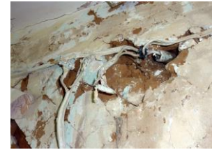
Lighting and power wiring!
